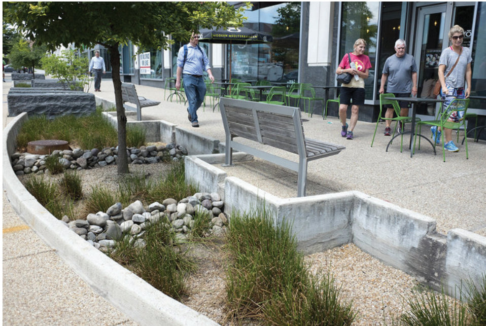
Cities are increasingly using green infrastructure, like this trench to collect rainwater, to better manage stormwater. The inlets on this trench are big enough to allow water to flow but small enough to prevent pedestrians from catching their feet in them. (David Kidd)
